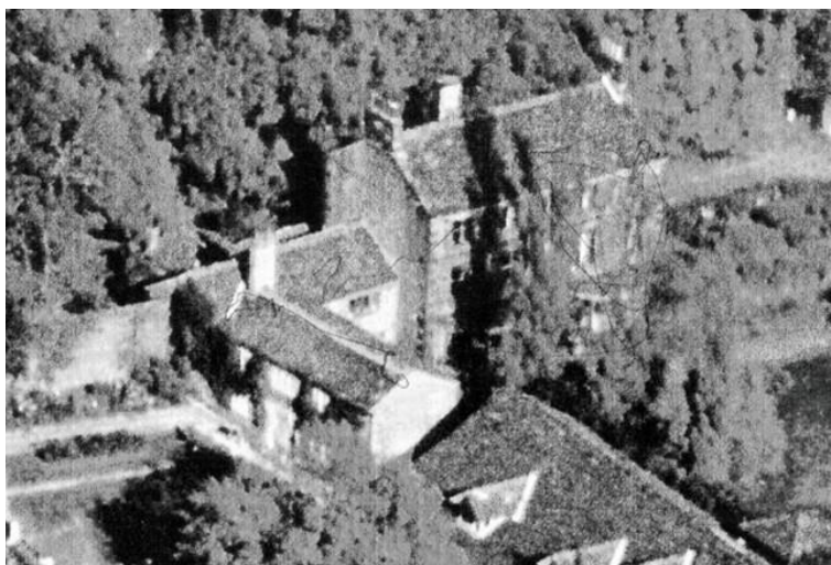
The now demolished Lightcliffe House
